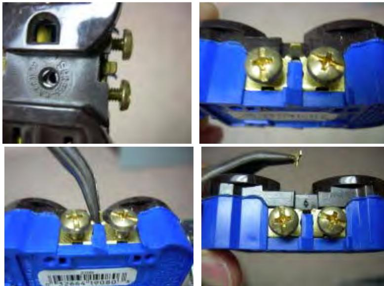
The first two graphics show the metal strip or tab. The third and fourth graphics show how the tab is easily removed with a set of needlenose pliers. Once the tab is removed, the upper and lower outlet plugs are independent so one can be, for example, controlled by a wall switch while the other is always on.
