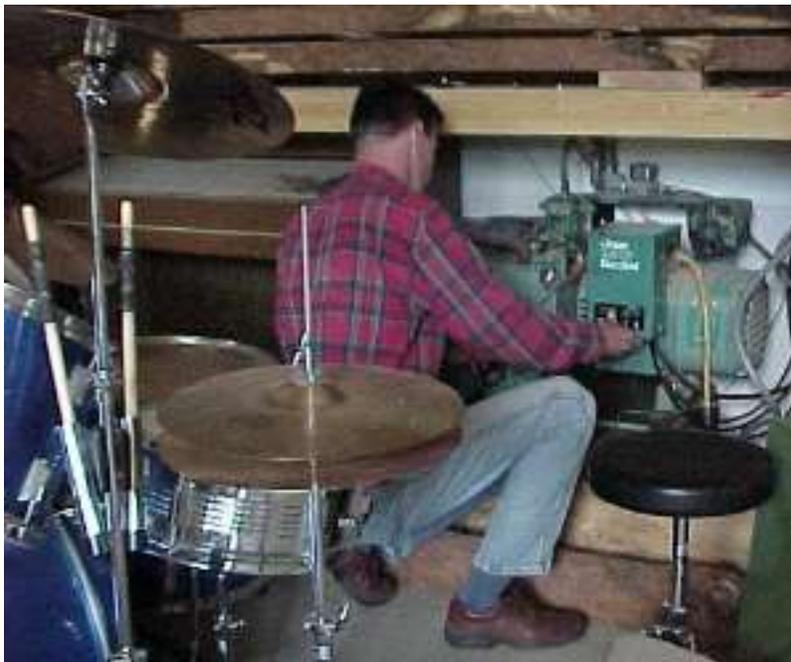
The generator's carburetor still functions in the normal way with this conversion, mixing air and fuel into the combustion chamber. You will need some special propane regulation and safety equipment, available from any generator shop that sells and services large propane generators (Onan, Kohler, Winco, etc.).
